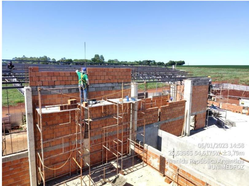
**Foto 25 – Alvenaria – Levante – Fachada Principal**
