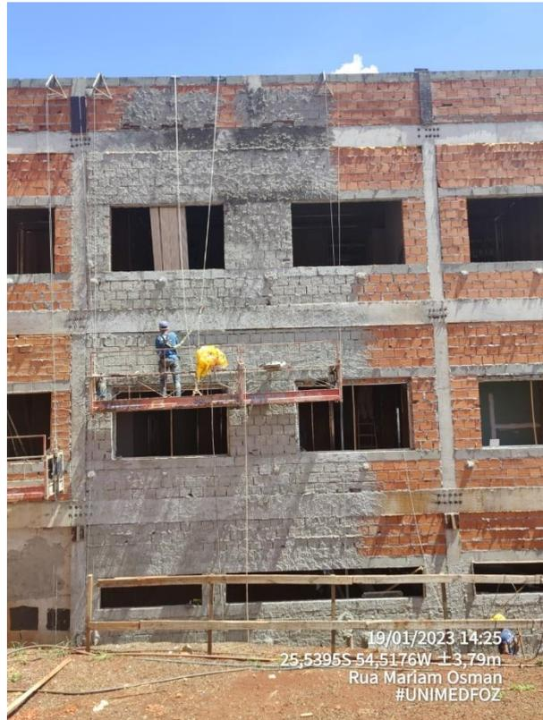
**Foto 27 – Alvenaria – Levante – Fachada Principal**
