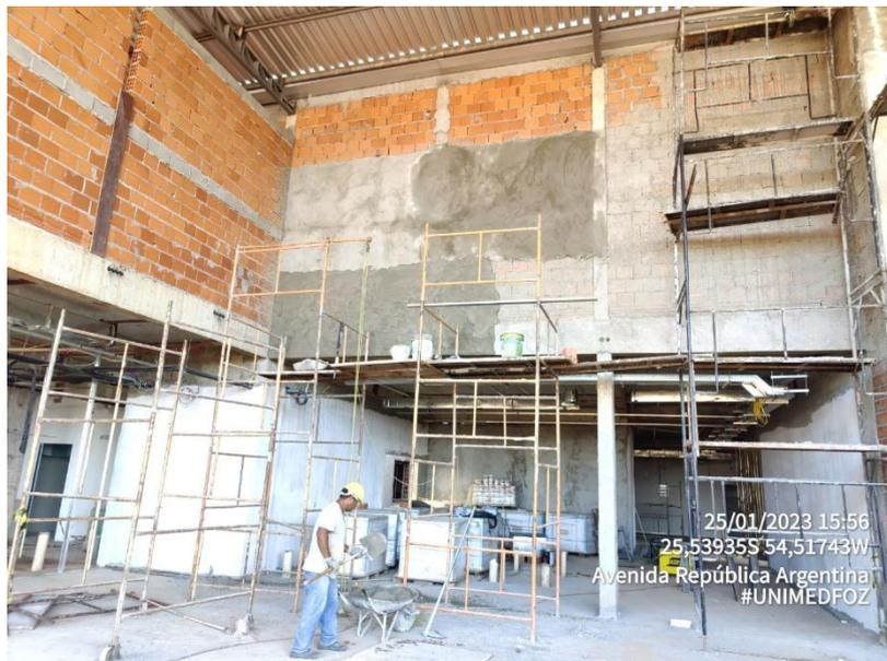
**Foto 28 – Alvenaria – Levante – Fachada Principal**
